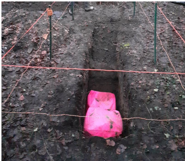
The ditch trench being dug out.
