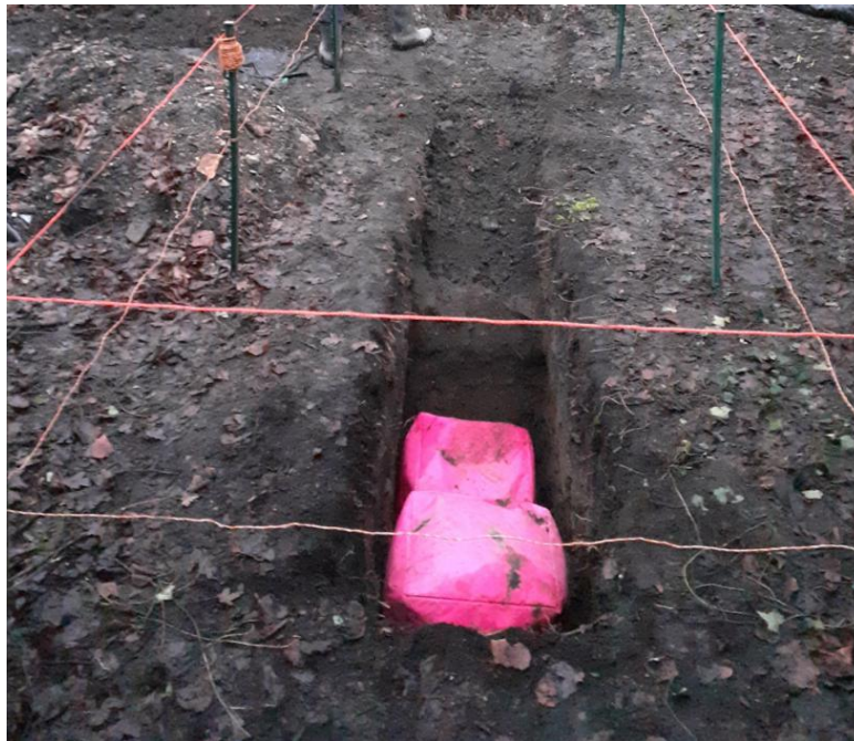
The ditch trench being dug out.
