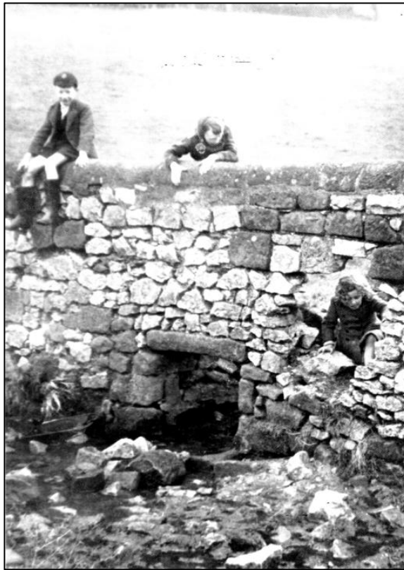
Bridge over the Yokecliffe Stream
